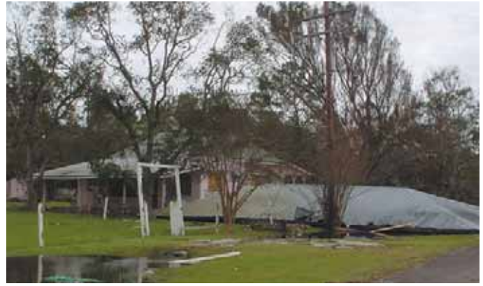
Here's the scene that Charles Wallace found after Hurricane Ike blew through his neighborhood. His neighbor's roof was resting on the lawn of Charles' flood-ravaged house.
